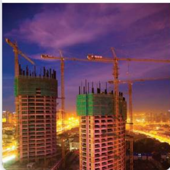
One of many construction sites in Beijing
